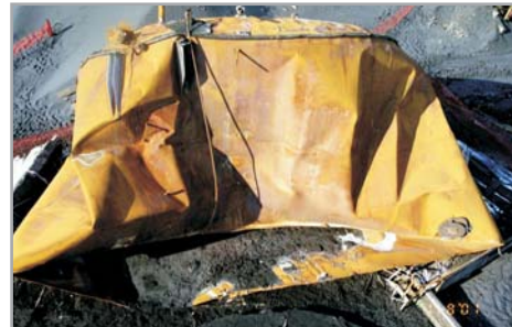
Collapsed Storage Tank
