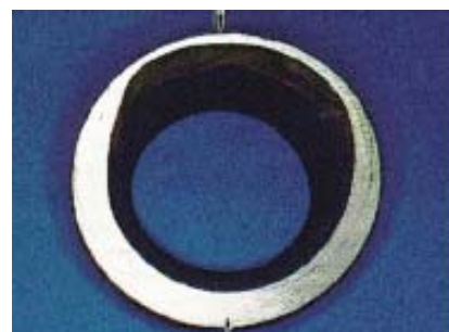
Internal wall thinning in a pipe subject to flow accelerated corrosion.
